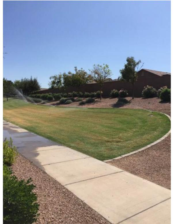
Dehydrated brown patches in turf and sprinkler puddles on sidewalk are signs of an irrigation system working inconsistently.
